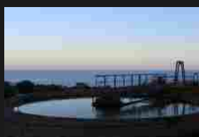
Telecontrollo Made in Italy
