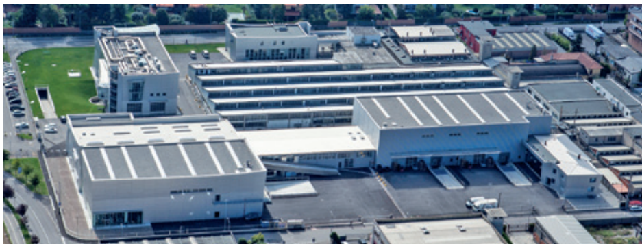
LOVATO Electric (Factory in Bergamo, Italy)
