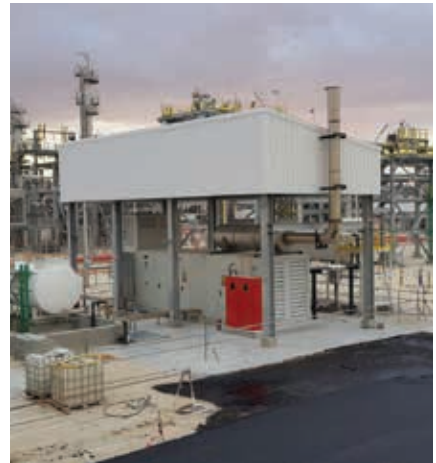
DGS for Oil& GAS applications, with CO 2 fire fighting system
