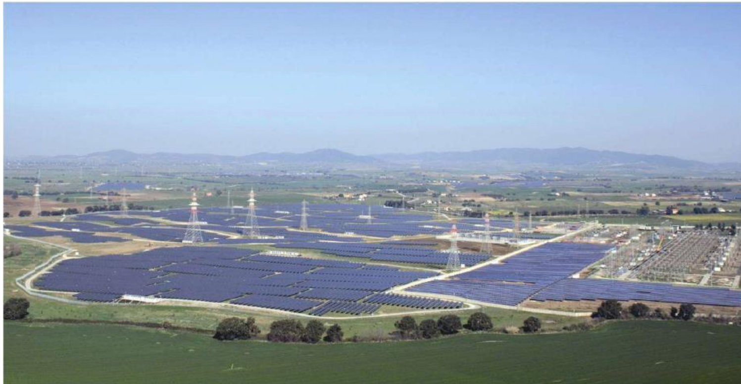
Montalto di Castro - ITALY - 84 MW powered with SMA Central Inverter
