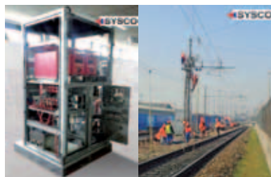
Installation team of Technological Plants, Electrical Panel and Converter
