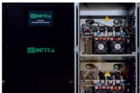
IVC Odyssey Turbo (SAG & SWELL compensator)
