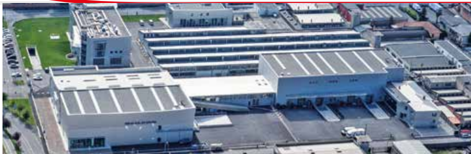
LOVATO Electric (Factory in Bergamo, Italy)
