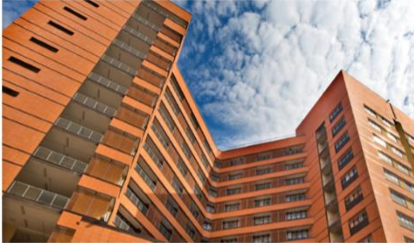
DEA Building 0 floor – tower B
