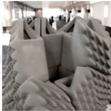
3D printed brick for the Quake Column designed by Emerging Object
