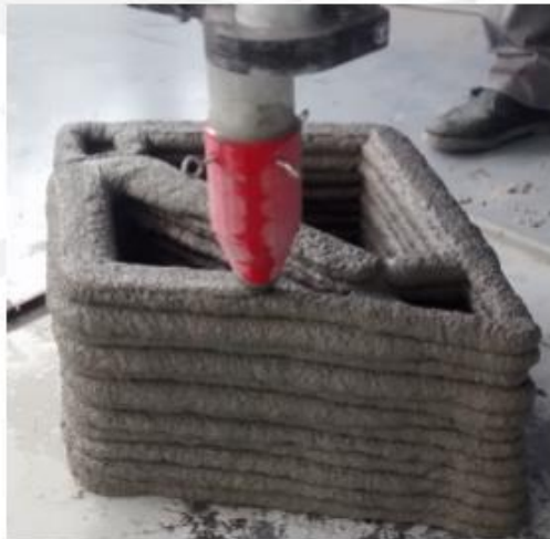
Concrete components 3D Printing
