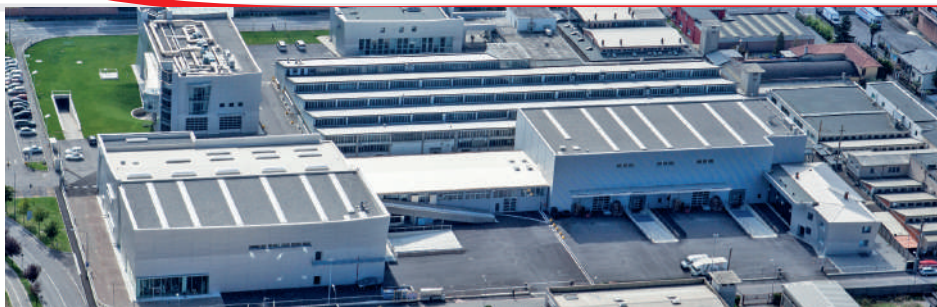
LOVATO Electric (Factory in Bergamo, Italy)
