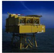
Borwin 1 400 MW HVDC
