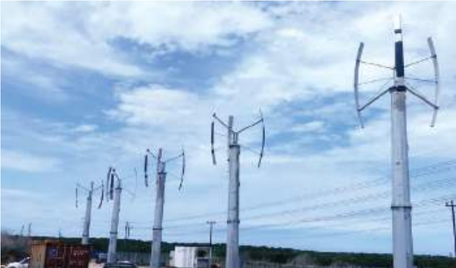
Minigrid with 5 10kw vertical axis wind turbine
