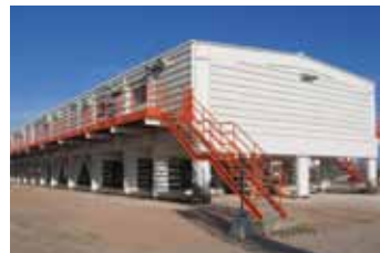
Local Equipment Rooms
