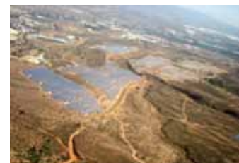
Almeria - Spain 10,8 MW on ground - 180Wp modules
